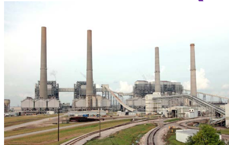
W.A. Parish Power Plant
